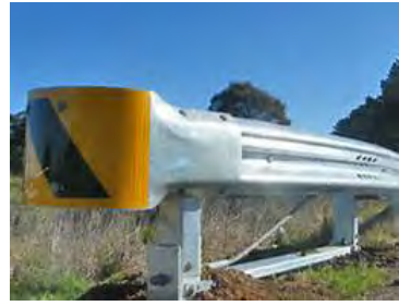
Modified Eccentric Loader Terminal
