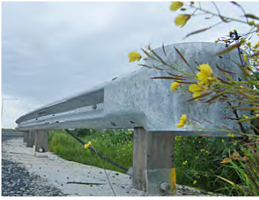
Breakaway Cable Terminal
