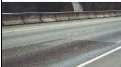
Chip Seal Repair Low
