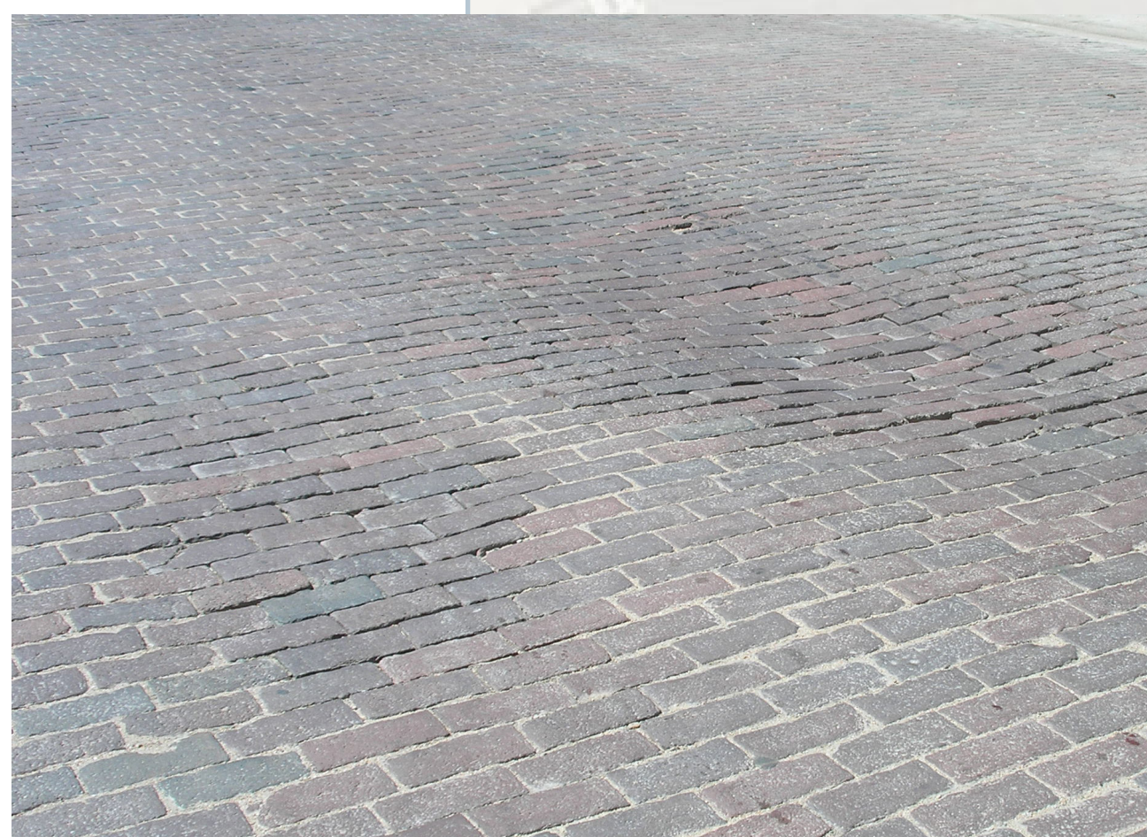
Horizontal/vertical displacement
