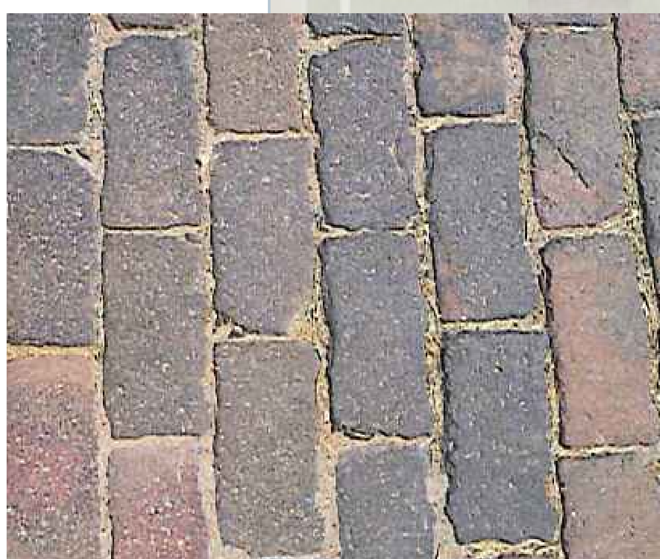
Corner breaks and rounded edges
